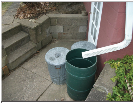
Rear Basement Door Area
