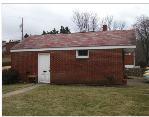
Garage Service Door
