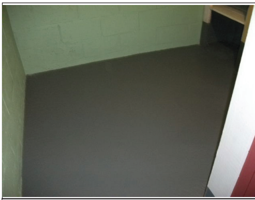
Open Basement Area
