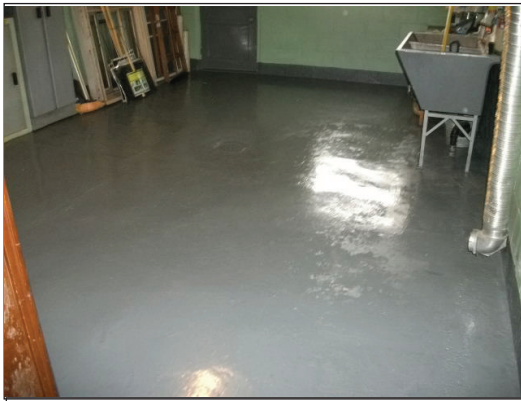
Open Basement Area
