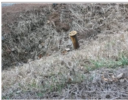
Meter Box Access Rear
