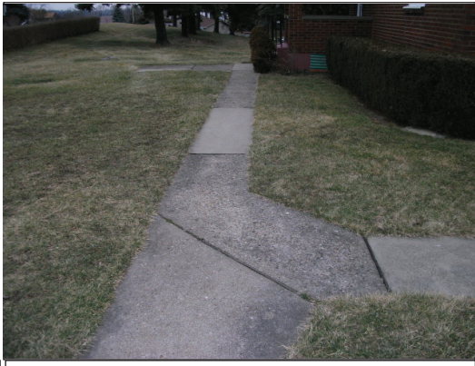
Typical Walkways Present
