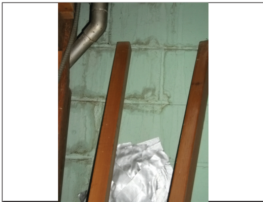
Mechanical Area Walls
