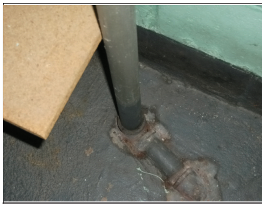
Gas Line Entrance Basement
