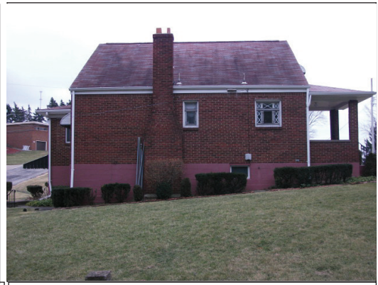
Rain Cap & Bird Screen Rec. To Chimney
