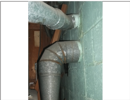
Flue for Furnace and HWT
